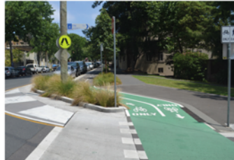
Separated bike lane intersection improvements
