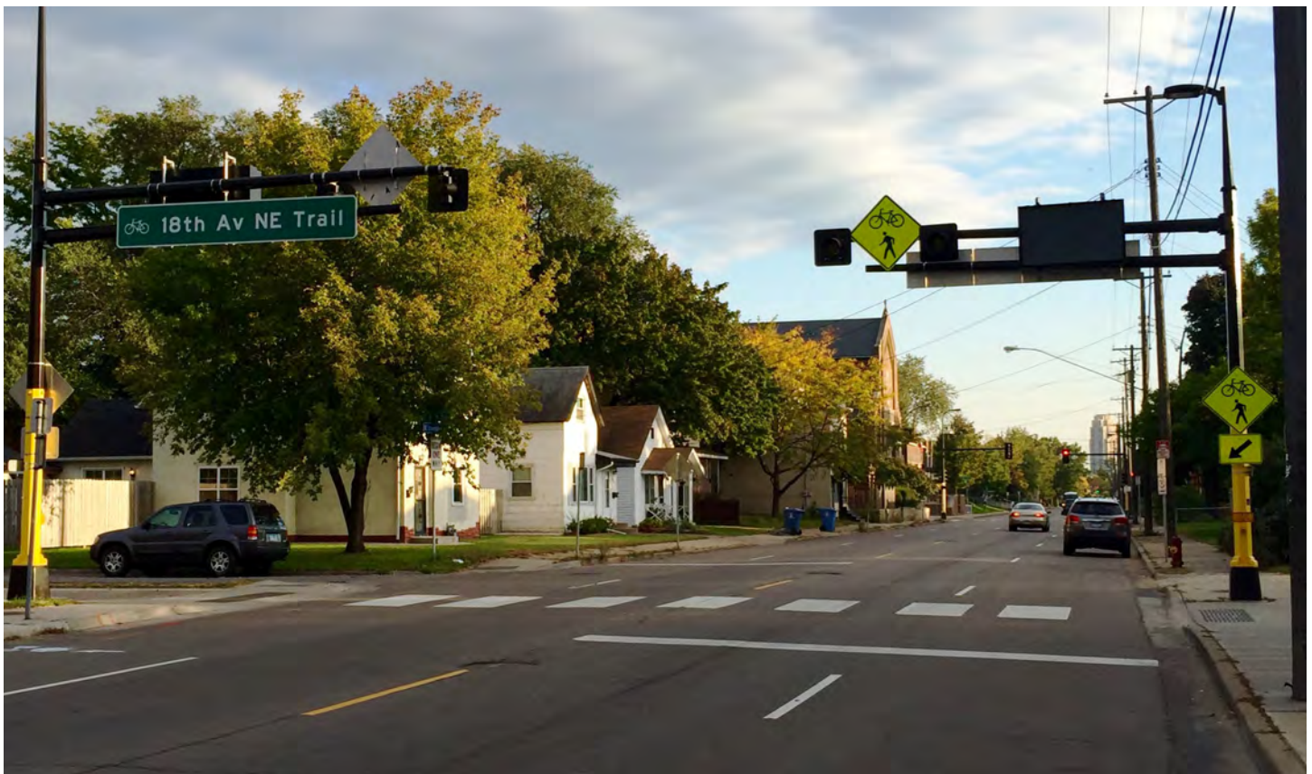
HAWK Signals increase safety for pedestrians and may be used for high volume crossings locations
