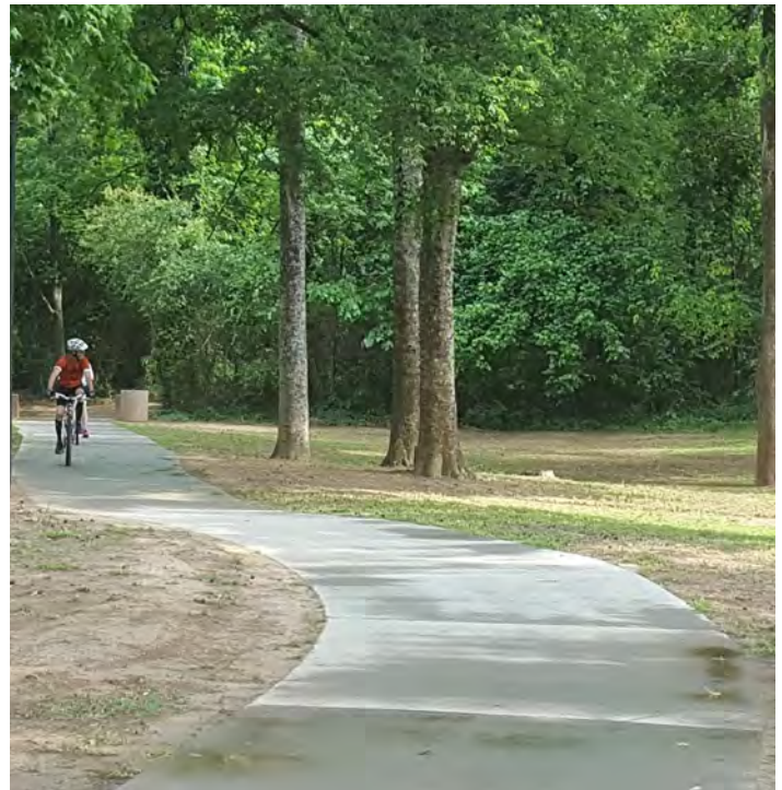
Three Rivers Greenway is an example of a LOC 1 facility
