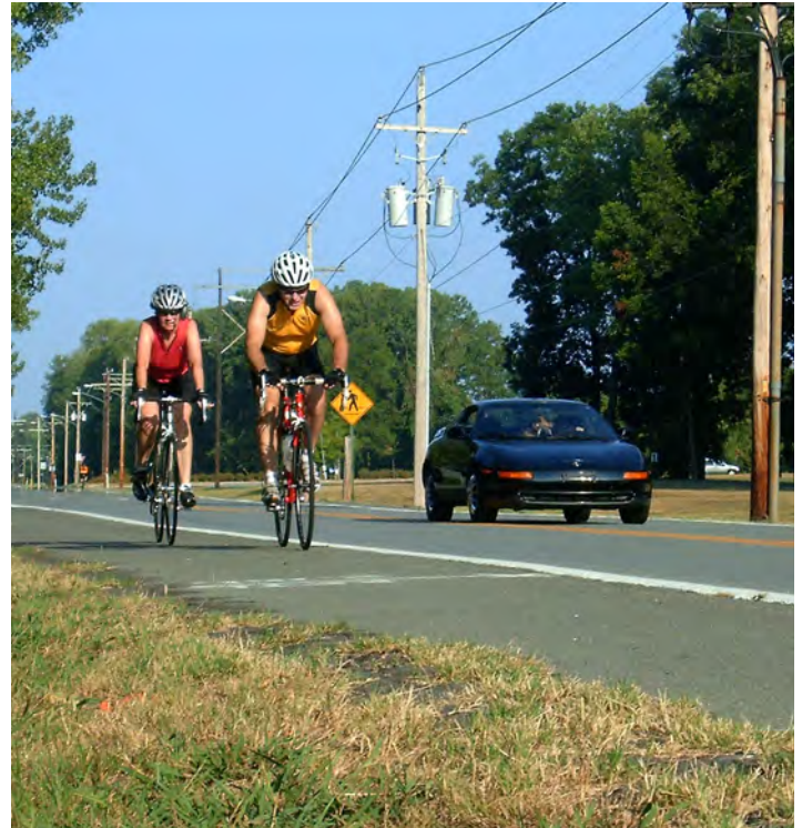
Paving shoulders on slower speed roads can create a more comfortable experience for cyclists
