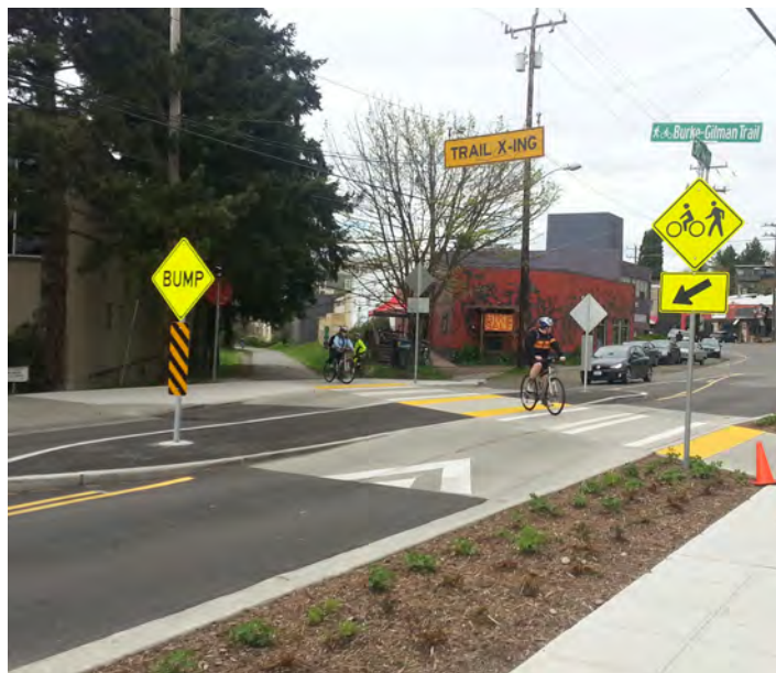
High visibility crossing are useful for mid-block trail crossing as well as downtown environments
