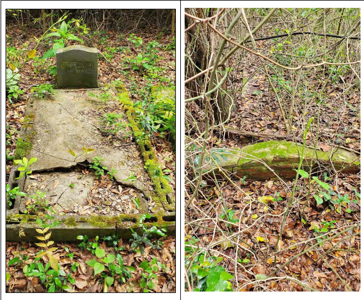
Figure 45. Grave of Emmanuel Hart with significant slab damage (left) and vault constructed grave damaged by tree growth (right).
