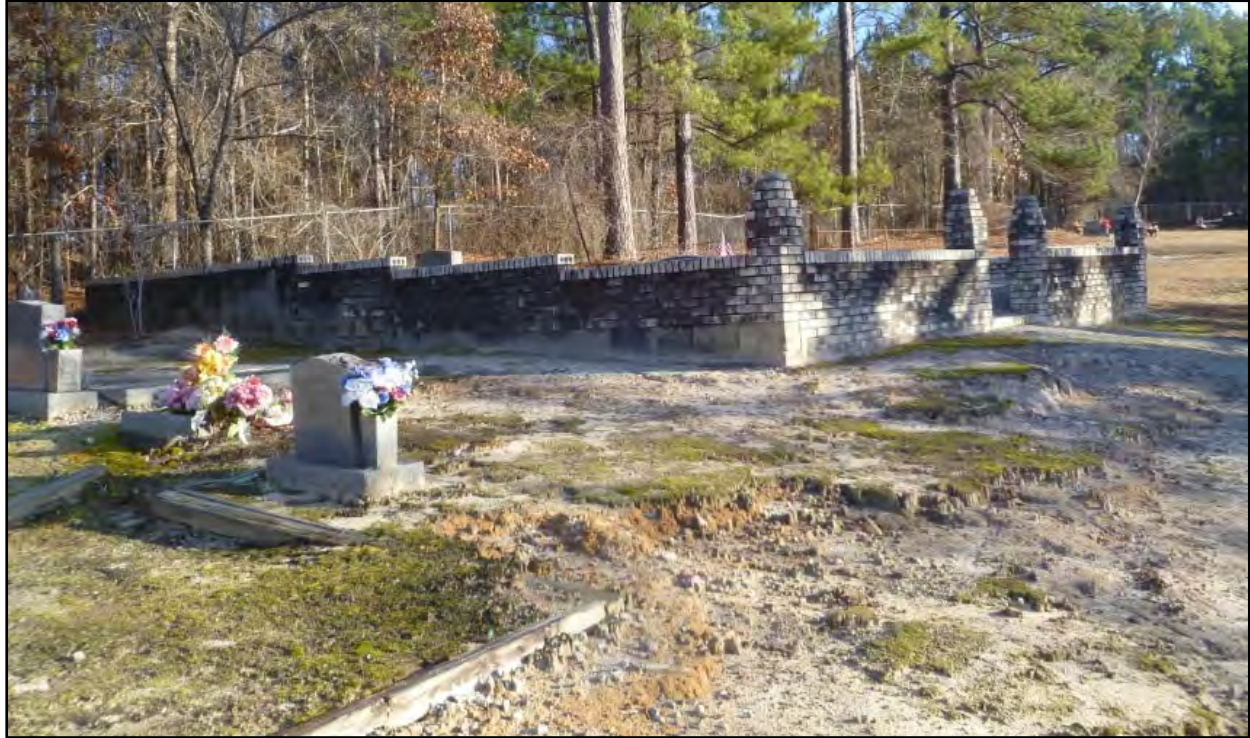
Figure 80. Example of erosion damage throughout Mt. Pisgah Cemetery.
