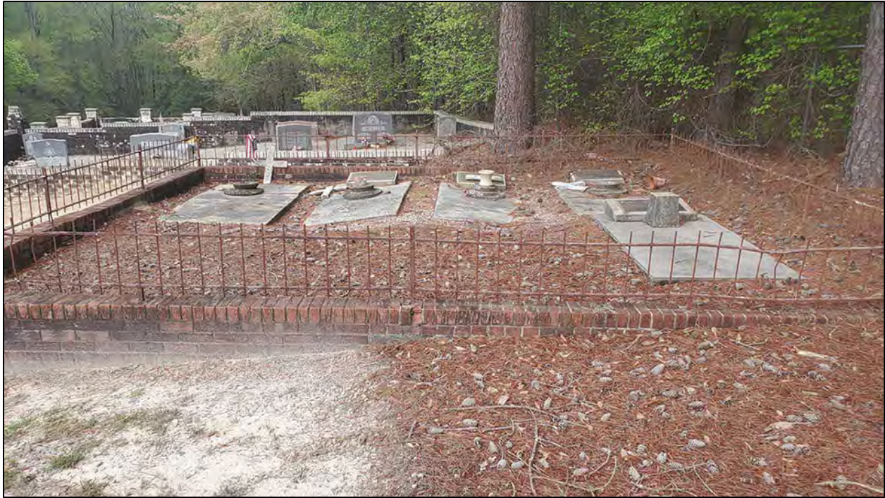
Figure 85. Jones Family plot showing shifting and broken ledgers.
