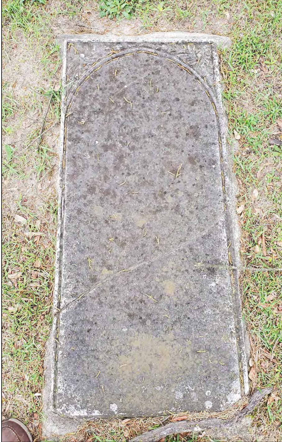
Figure 105. Headstone of Keziah Arthur set horizontally and exhibiting cracking.
